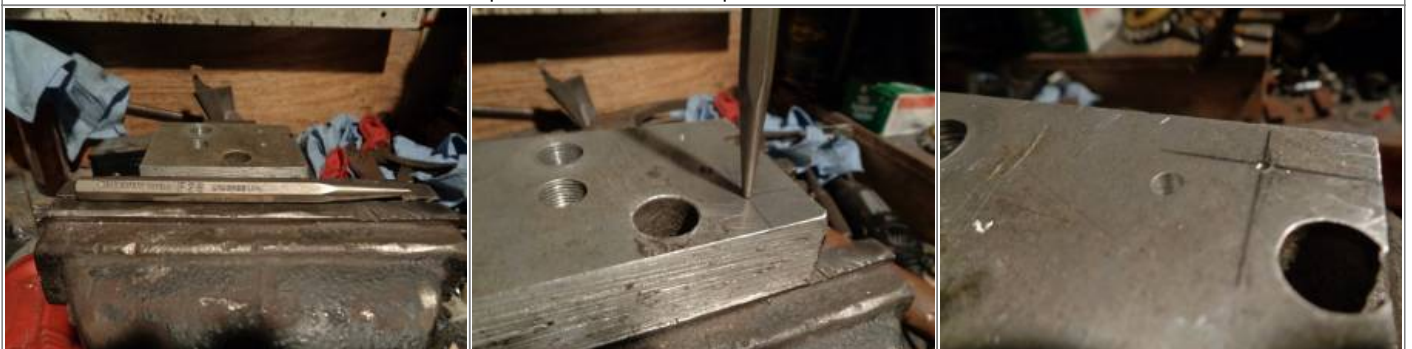
Center punch used to make a pilot hole for the drill bit. 5)
